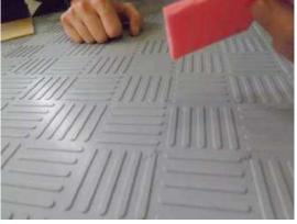
13. You can scrape off excess with flat scraper and some acetone if necessary
