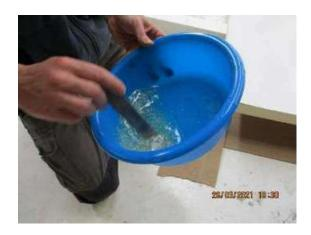
3. Pour in the peroxide (between 1.5% and 2% maximum) in the resin + fiberglass mixture and mix  $\frac{1}{2}$
