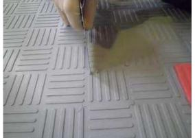
9. Position the mould using the markers you have made
